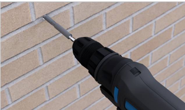
Screw the stud screw into the brick wall.
