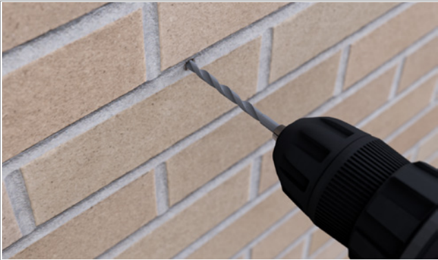
Drill -slightly inclined upwards- an 8 mm hole in the joint for the pin.
